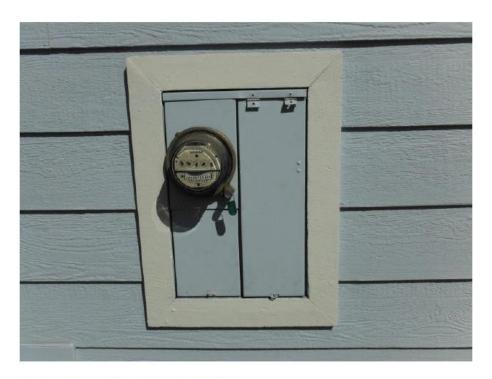
703 SERVICE RATING 120/240 volt system, rated at 100 Amperes.
